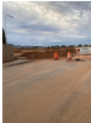
Areas on Village Dr. that require maintenance and remediation. Gutter flow line, Stockpile at intersection at utility connection and North side of site entrance; all presenting sediment pollution movement from project.
