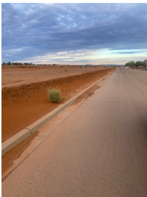
Areas on Village Dr. that require maintenance and remediation. Gutter flow line, Stockpile at intersection at utility connection and North side of site entrance; all presenting sediment pollution movement from project.
