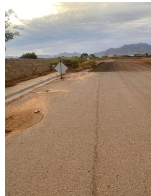
Areas on Village Dr. that require maintenance and remediation. Gutter flow line, Stockpile at intersection at utility connection and North side of site entrance; all presenting sediment pollution movement from project.
