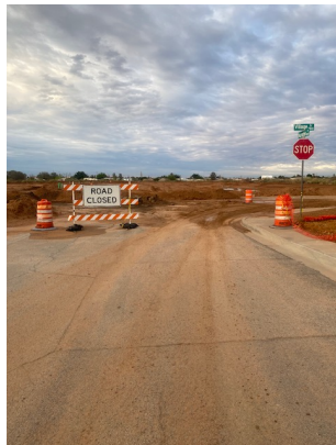
Areas on Village Dr. that require maintenance and remediation. Gutter flow line, Stockpile at intersection at utility connection and North side of site entrance; all presenting sediment pollution movement from project.
