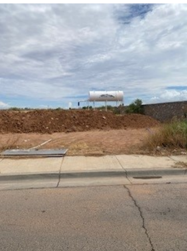
Significant sediment tracking and deposition on Village Drive
