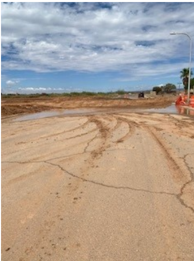
Significant sediment tracking and deposition on Village Drive
