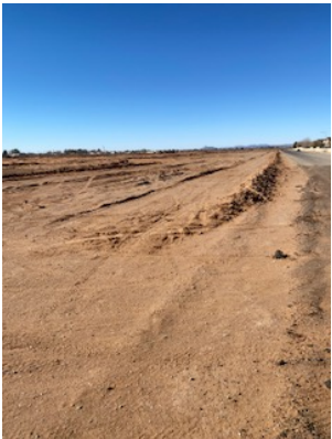
Erosion control berm along North perimeter
