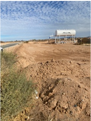
Erosion control berm at South West water tank area
